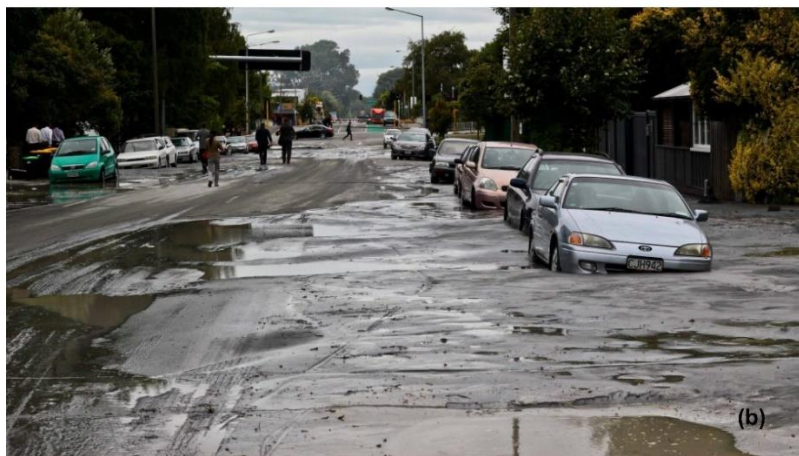
Figure 1-1: (a) Liquefaction-induced foundation failure of Kawagishi-cho apartment buildings during the 1964 Niigata earthquake (Source: Kramer [22]) and (b) consequences of liquefaction following the 2011 Christchurch earthquake in New Zealand (Source: www.geotech.hr ).
