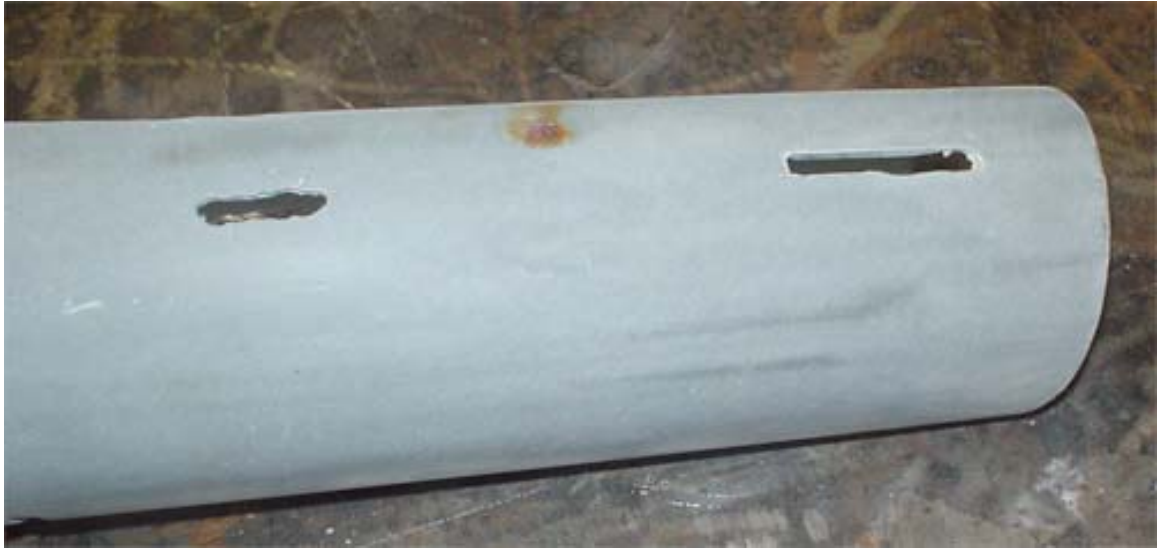
Figure 3.16- Holes made for straps
