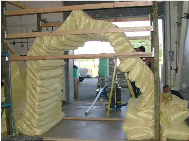
Figure 66. Air-Filled 46 Bag Structure, 5 pipes guiding bag filling.
