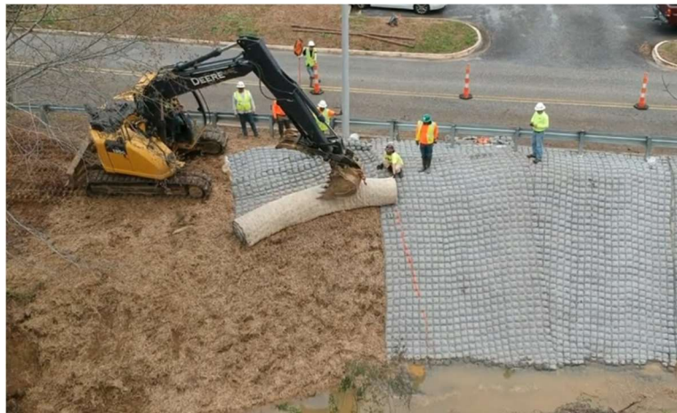
Figure 5: Example of Field Installation of Block Mats (Motz Enterprises, Inc., 2021)
