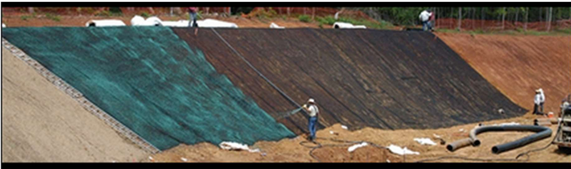
Figure 8: TRM Installed in Practice (Tenax US, 2021)
