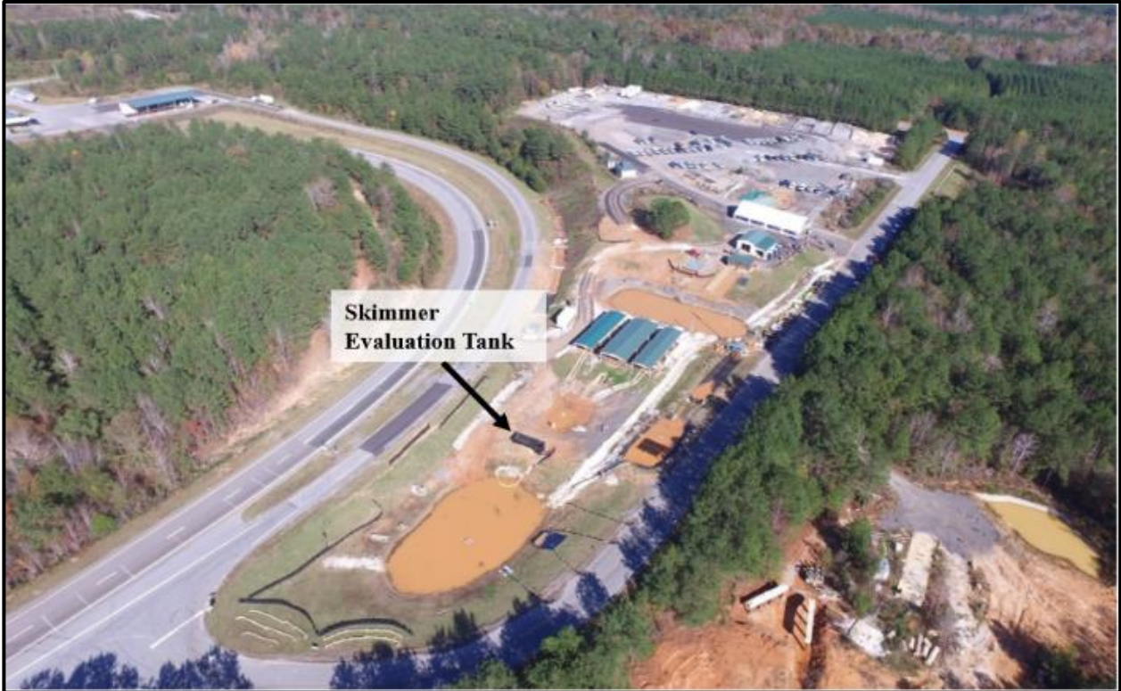
Figure 16 Skimmer Evaluation Tank at AU-SRF.
