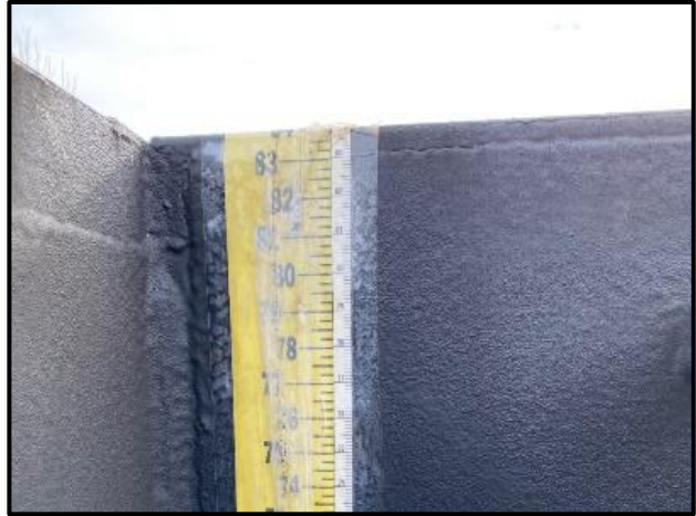
(b) Tape measure adhered to tank wall
