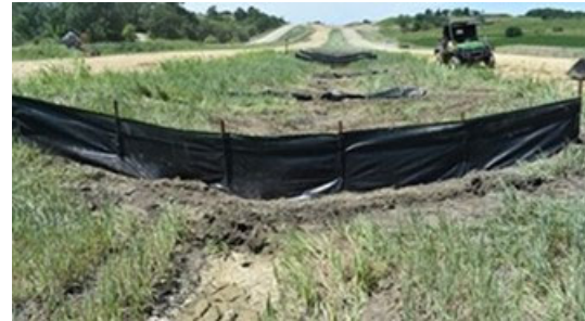
(b) SF-S field installation
