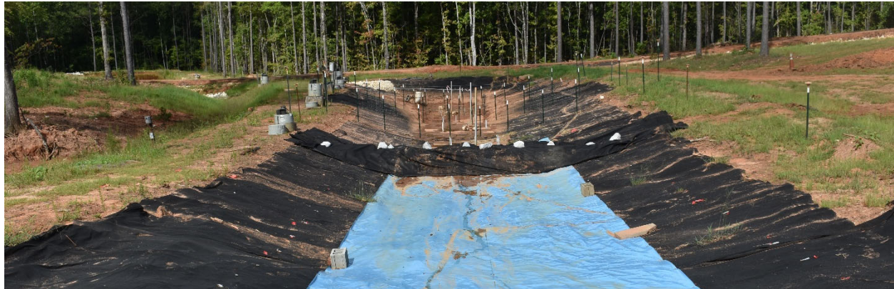
(a) forebay installation
