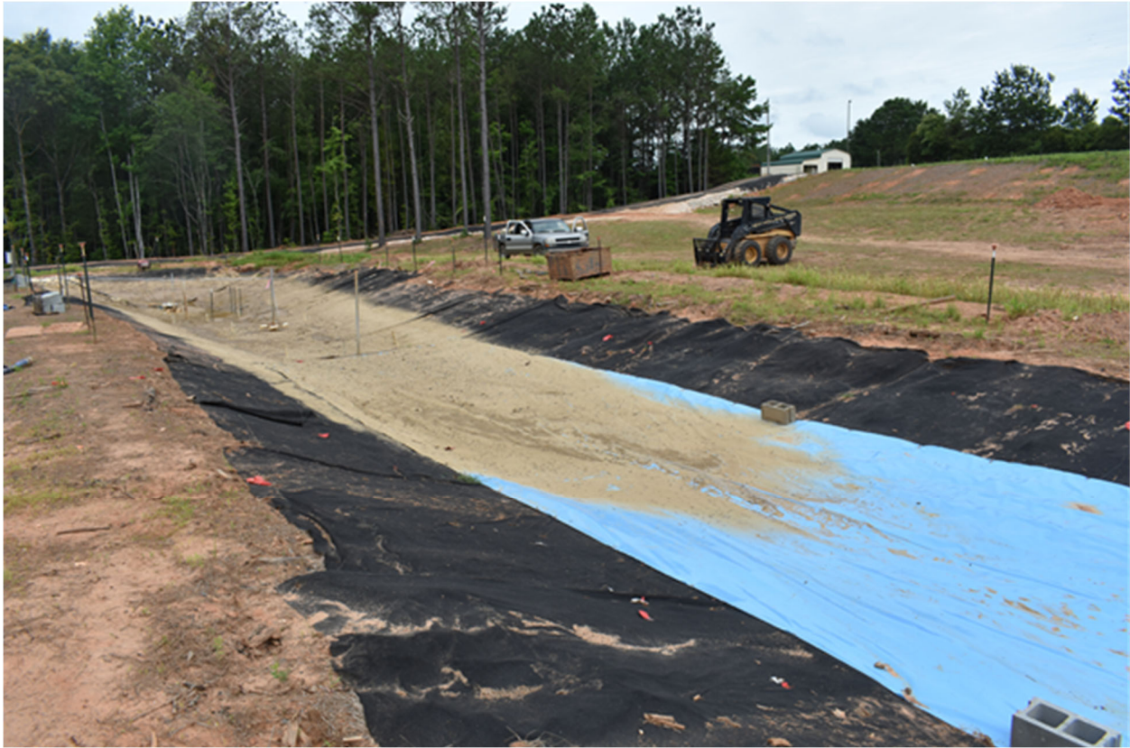
Figure 4.25. In-channel sedimentation due to skimmer installation.
