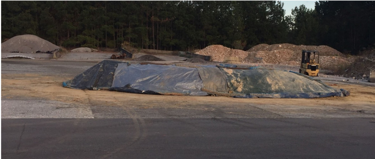
(b) compacted and covered stockpile
