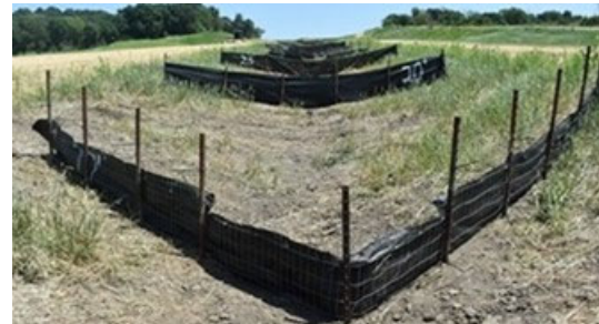
(f) SF-M2 field installation
