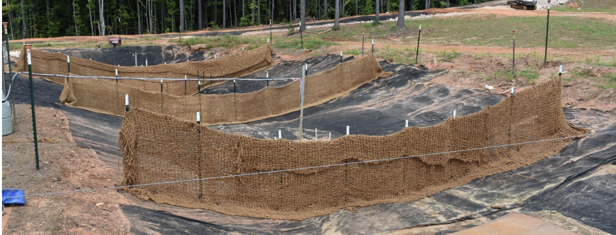
(a) coir baffles after install
