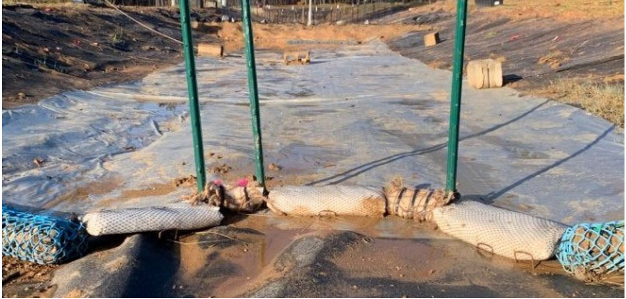
(a) placement in channel
