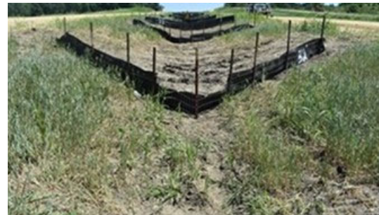
(h) SF-M3 field installation
