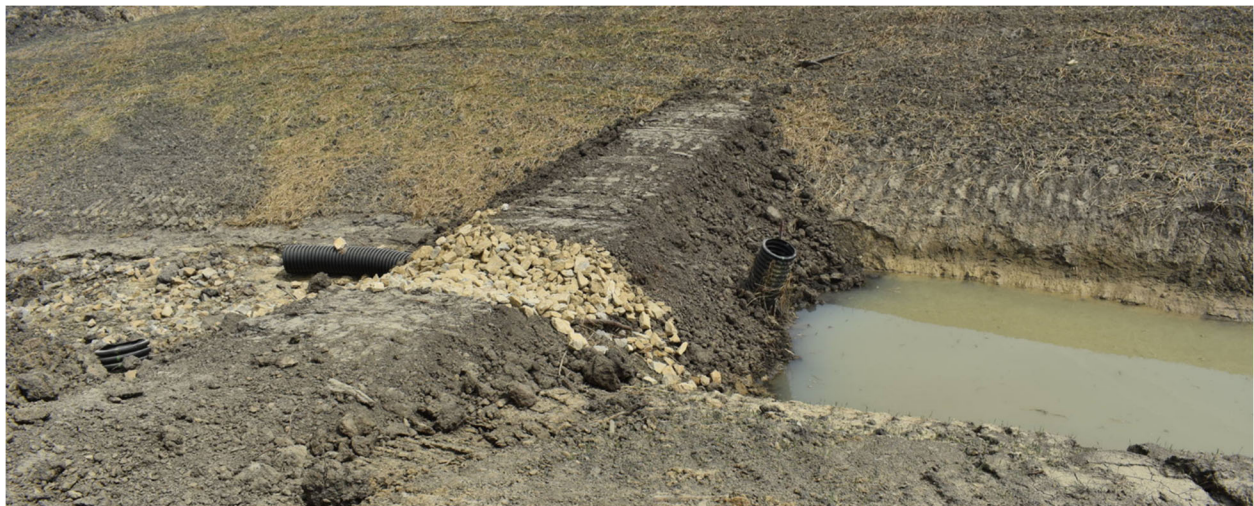
(a) Iowa DOT sediment basin installation
