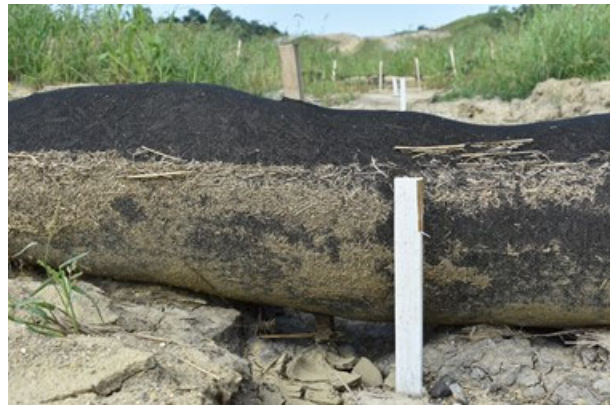
(c) stake shown on wattle after undercutting
