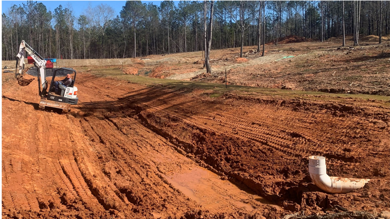
(a) channel grading
