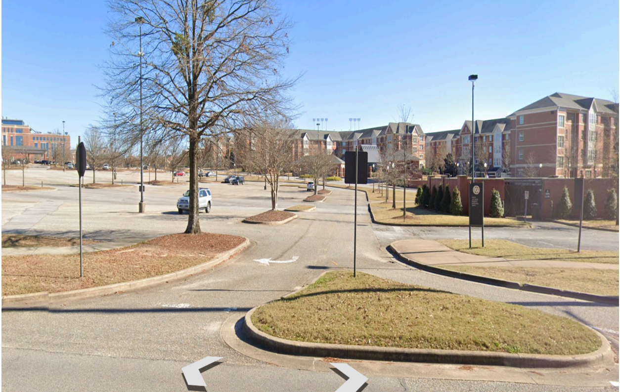
Figure 15 Ground view of Wire Road at the Entrance near War Eagle Way (27)
