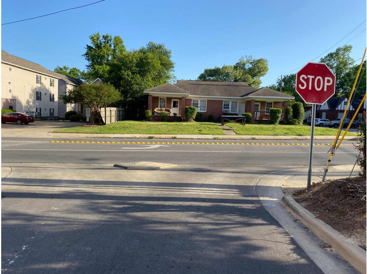
Figure 11 Alternate Ground view of Glenn Avenue at the Apartment Entrance
