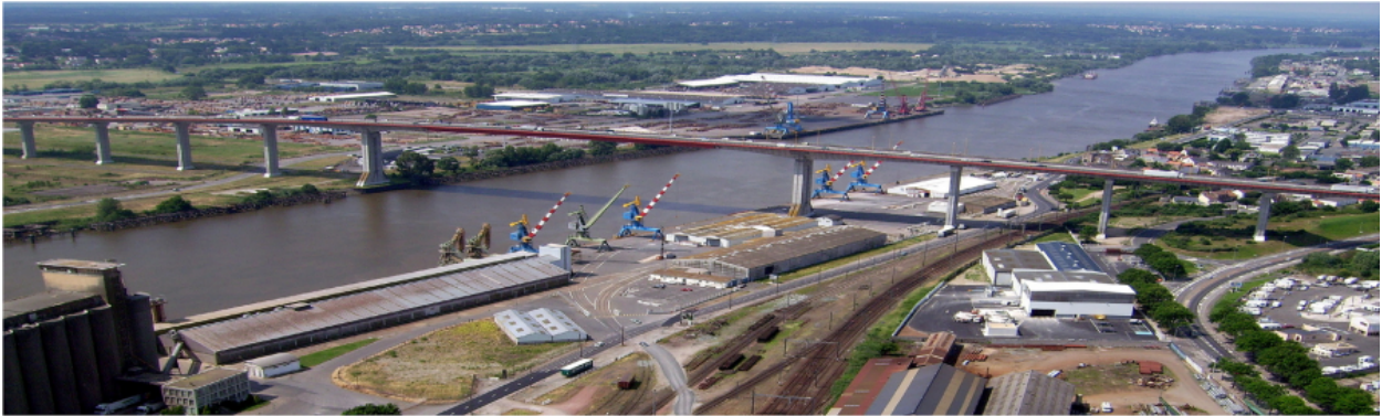
Figure 2-19: Bridge of Cheviré in France
