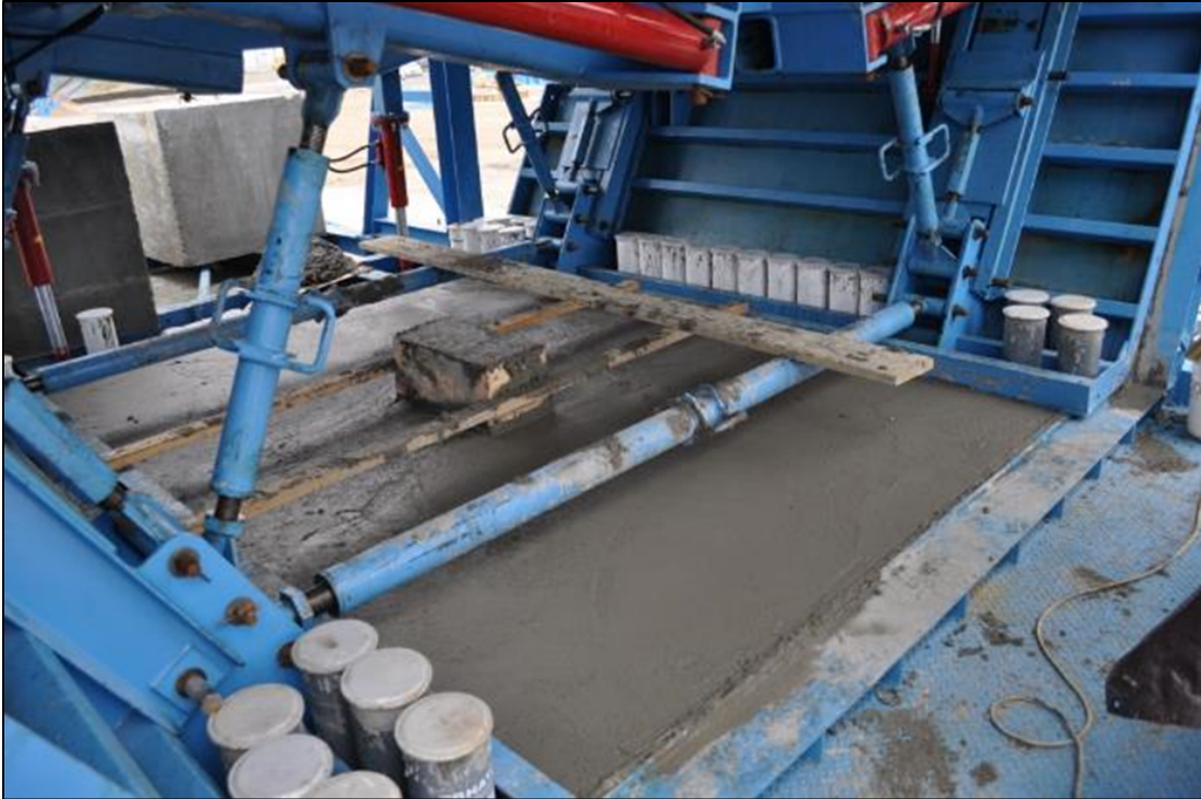
Figure 4-4: Placement of test specimens in segment forms for field curing
