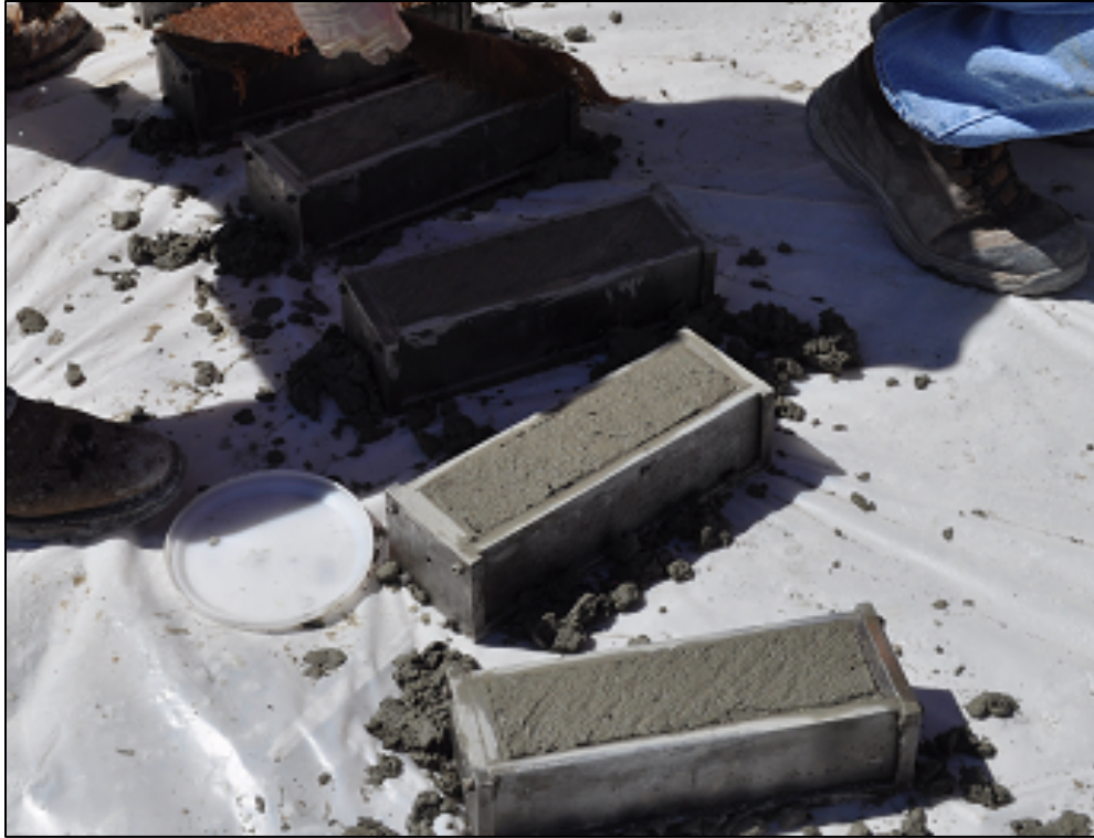
Figure 4-3: Preparation of concrete prisms on the jobsite
