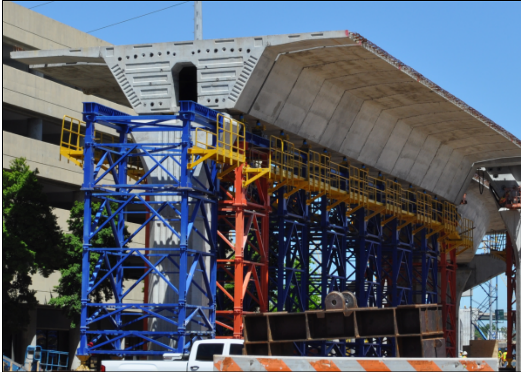
Figure 1-2: Birmingham I-59/I-20 segmental bridge during construction
