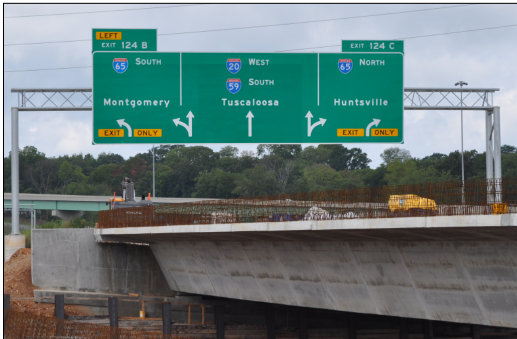
Figure 1-1: Birmingham I-59/I-20 segmental bridge during construction
