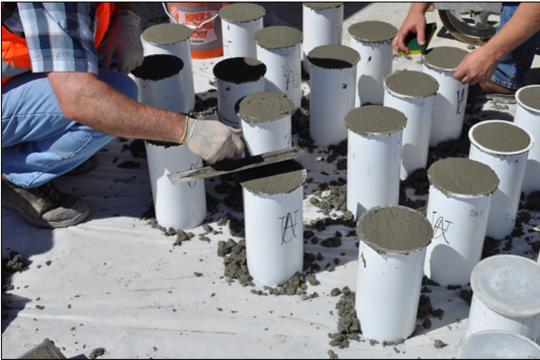
Figure 4-2: Preparation of concrete cylinders on the jobsite
