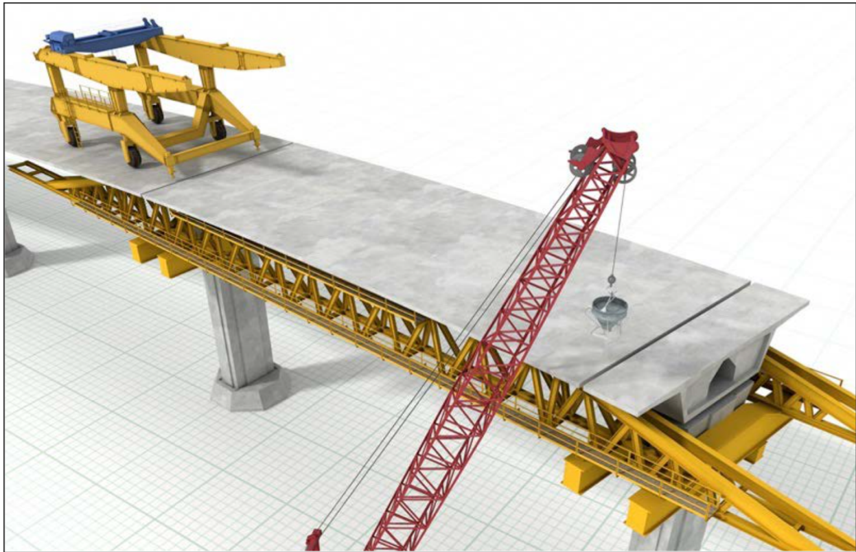
Figure 2-12: Cast-in-place closure joint (ASBI 2019)
