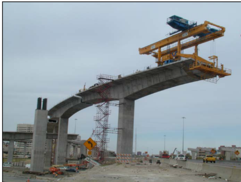
Figure 2-15: Balanced cantilever construction using mobile lifter (ASBI 2019)
