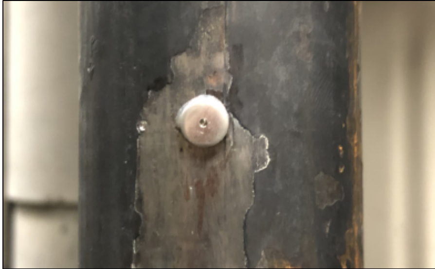
Figure 4-15: DEMEC point epoxied to steel rod for monitoring load
