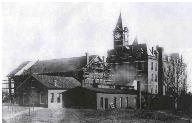
Langdon Hall during construction. Image courtesy of Auburn University
