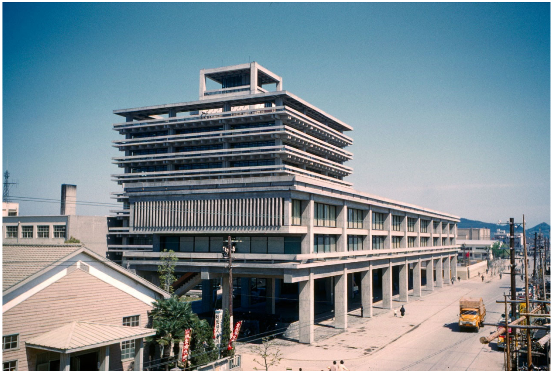
Figure 51: Communications Centre in Kofu (Tange, 1962)
