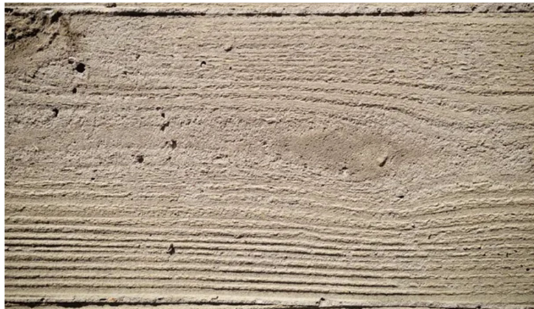
Figure 73: Cast Concrete Texture ( Wood Grain Left in a Concrete Wall | GL Barnhart Construction ...The Blog, n.d. )
