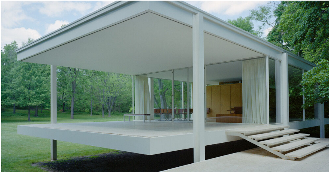
Figure 29: Farnsworth House, Plano, Illinois, U.S. (Rohe, 1945)
