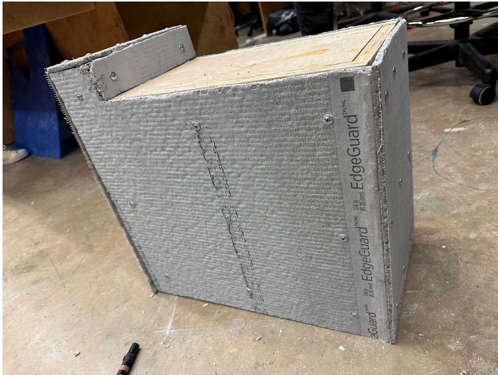
Figure 96: Attaching Cement Board.
