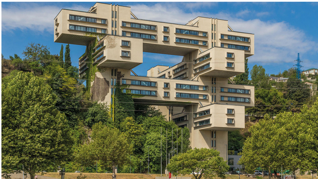
Figure 43:Bank of Georgia (Chakhava, 1975)
