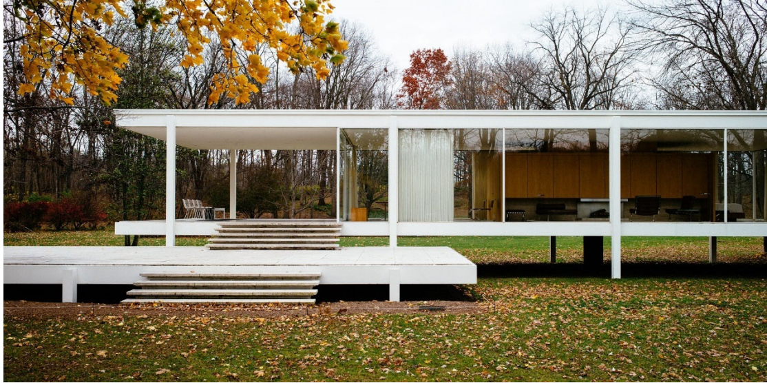
Figure 28: Farnsworth House, Plano, Illinois, U.S. (Rohe, 1945)
