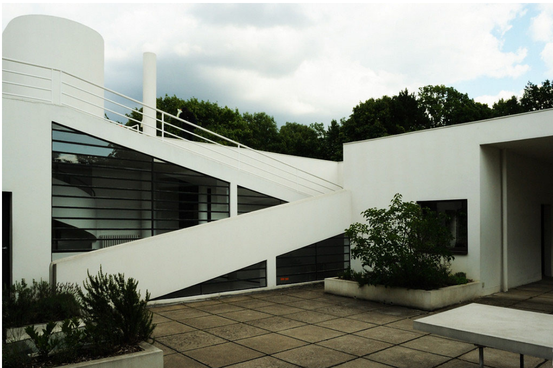
Figure 26: Villa Savoye Stairs (Corbusier, 1931).
