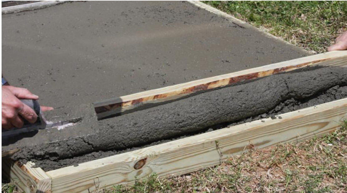
Figure 69: Pouring Cement (Gage, 2018).
