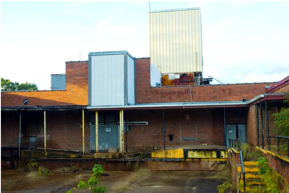
FIGURE 28: Abandoned plant in Hale County 2 (Smith, 2006)
