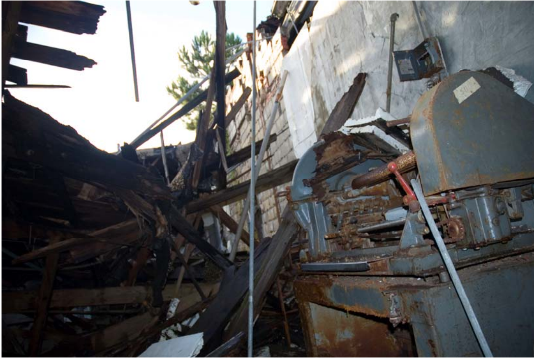
FIGURE 29: Abandoned plant in Hale County 3 (Smith, 2006)
